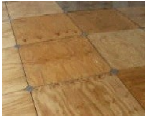
Laydown Plywood Flooring
