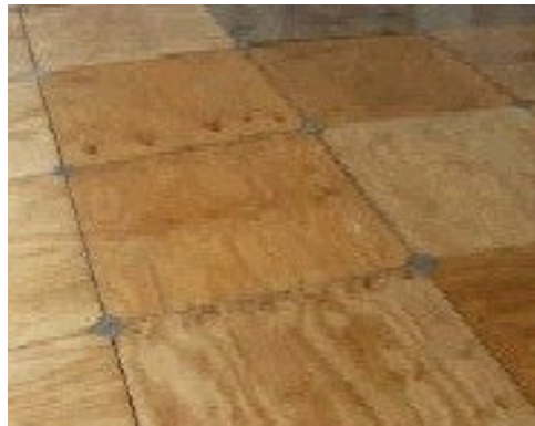
Laydown Plywood Flooring
